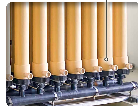
Hollow fiber membrane modules
